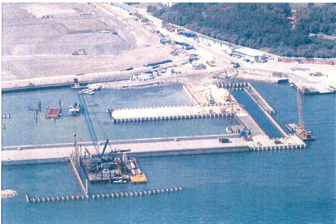
FIG. 1.1 - LAVORI ALLA CONCA DI MALAMOCCHO (2007) – ALLOGGIAMENTO PORTA LATO LAGUNA
