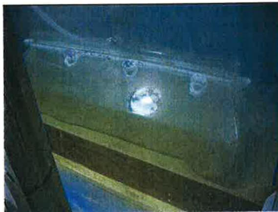
Figure 15 sand entrained into the caisson compartment under the side wall (Series 1)
