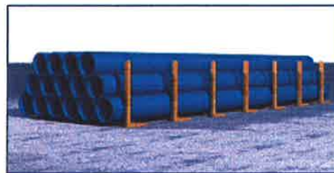
Figure 32. Loose Pipe Storage
